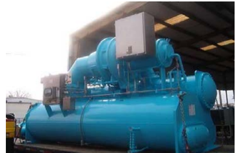
Trane Model CVHF W/C Centrifugal Chiller AFTER
