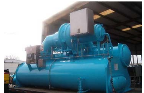
Trane Model CVHF W/C Centrifugal Chiller AFTER
